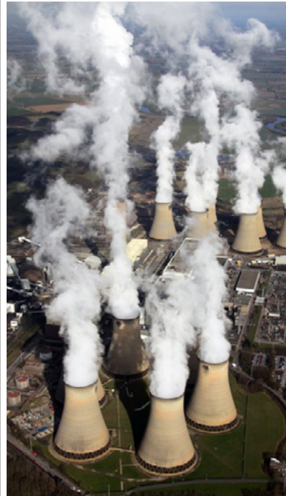
Drax Power Station
